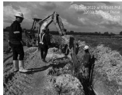
Earthing works and cable laying works
