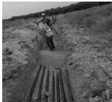
Earthing works and cable laying works
