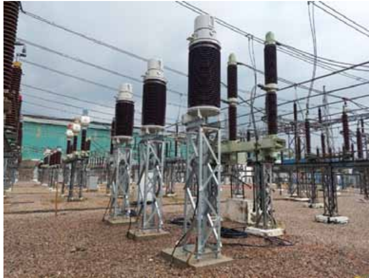
Primary bay of substation
