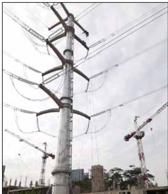
Monopole pylon towers
