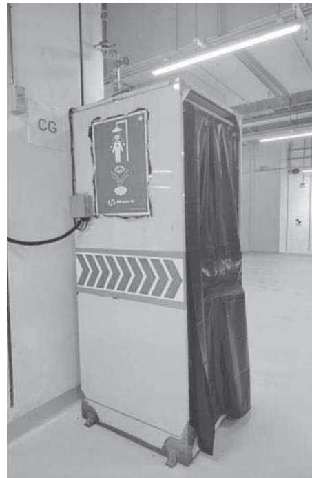
An eyewash station installed at one of our projects
