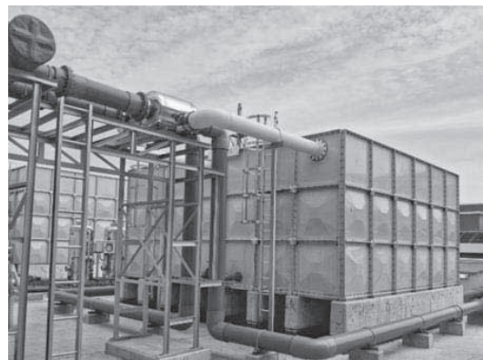
A rainwater harvesting system that we installed with retention tanks and drainage pipes
