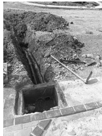
Underground telecommunication pipe and pit
