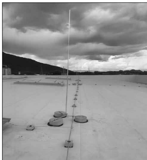
Lightning protection system
