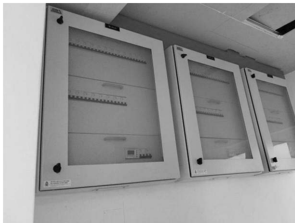
Isolated power supply
