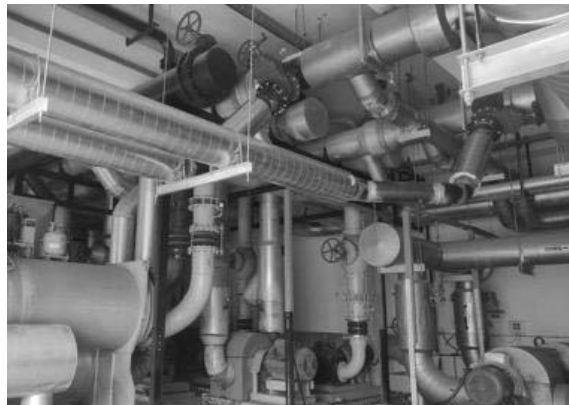
Water-cooled chiller system
