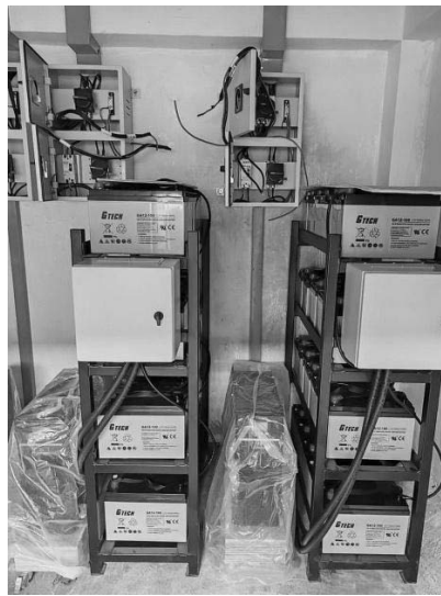
Uninterruptible power supply
