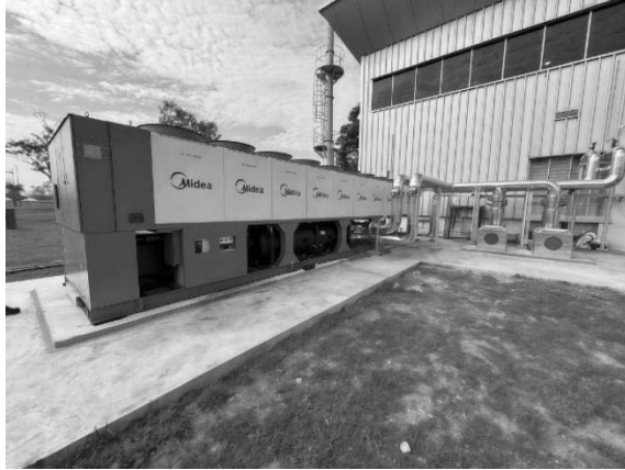
Air-cooled chiller system
