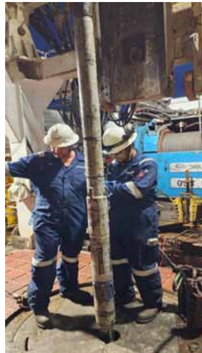
Section milling operation
